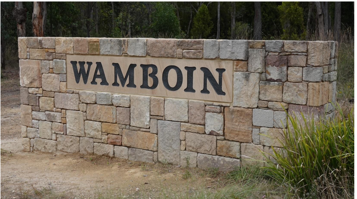
Below: The completed, restored entrance sign
